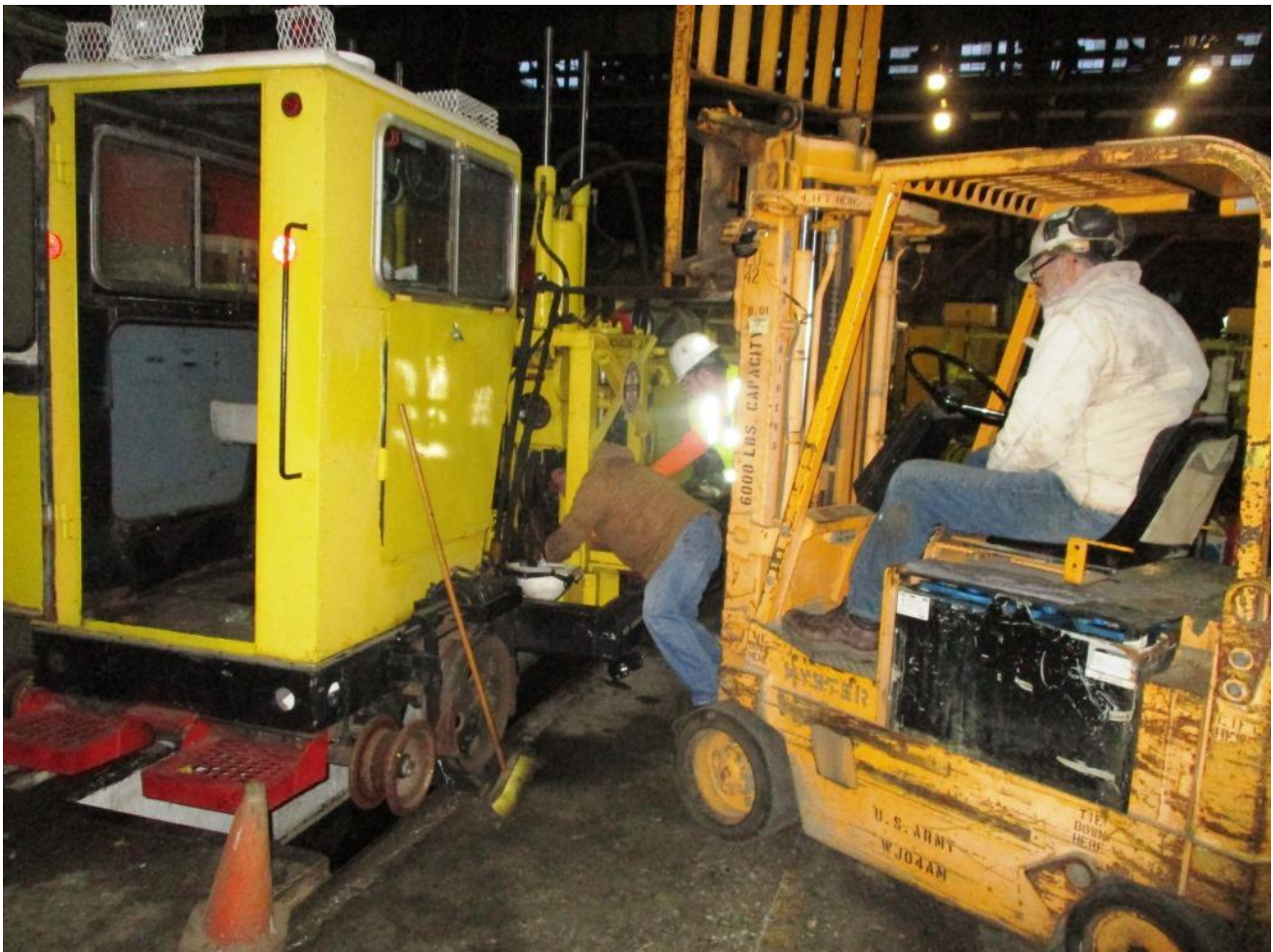
With Alan on the forklift supporting the cylinder, Mike H. and Chris H. work on removing the pin holding the cylinder in place
