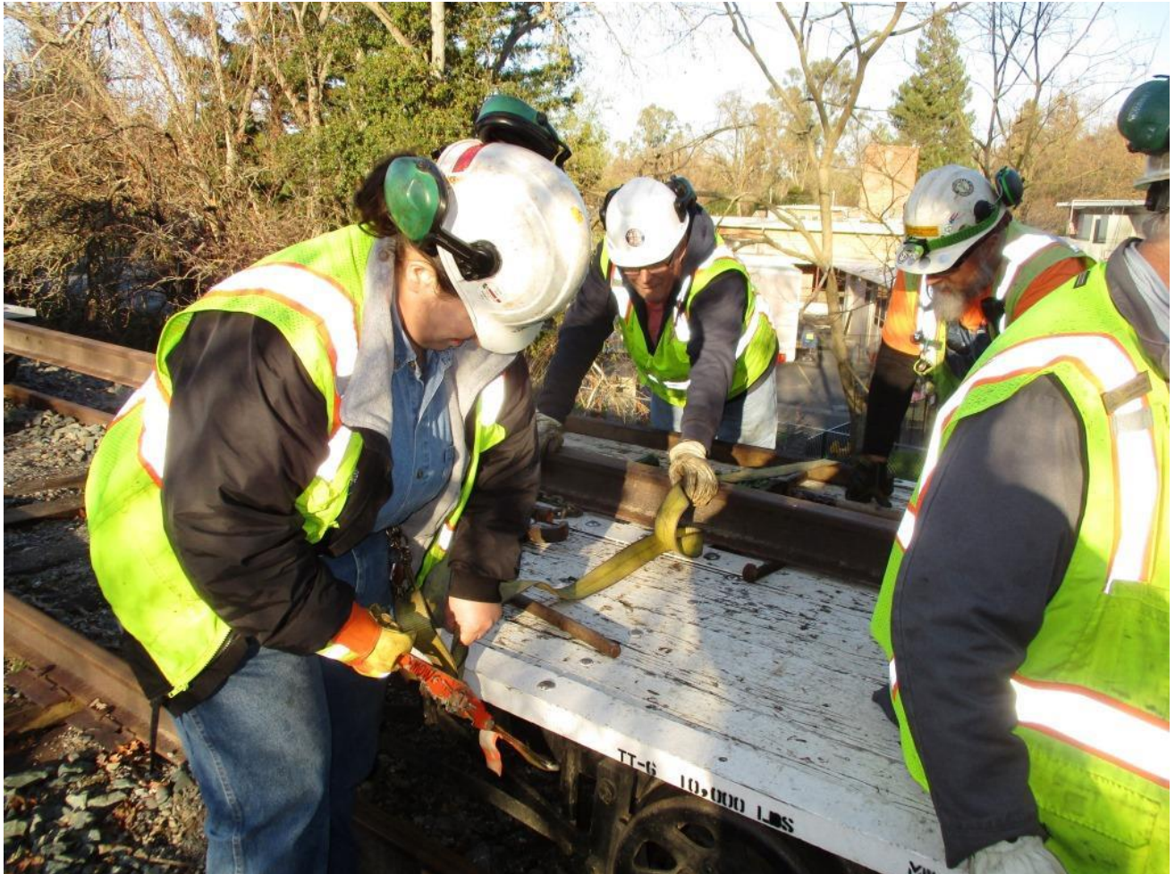
Heather, Bill, and Mike F. secure the rail to the flatcar with a strap
