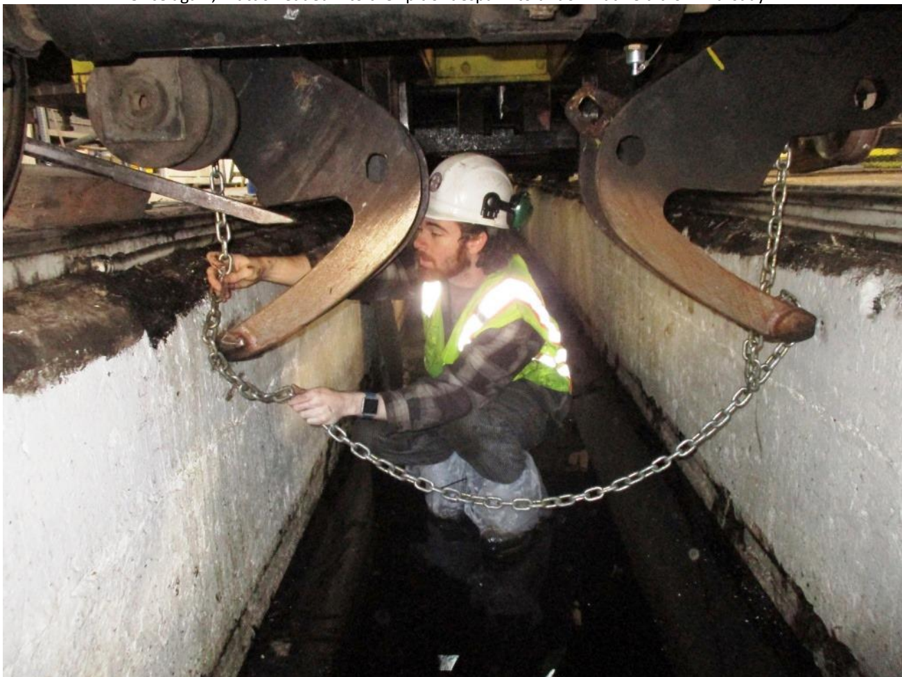
...Because the kickers needed to be dropped to remove an extraneous piece of metal (kicker on the right) preventing it from raising all the way
