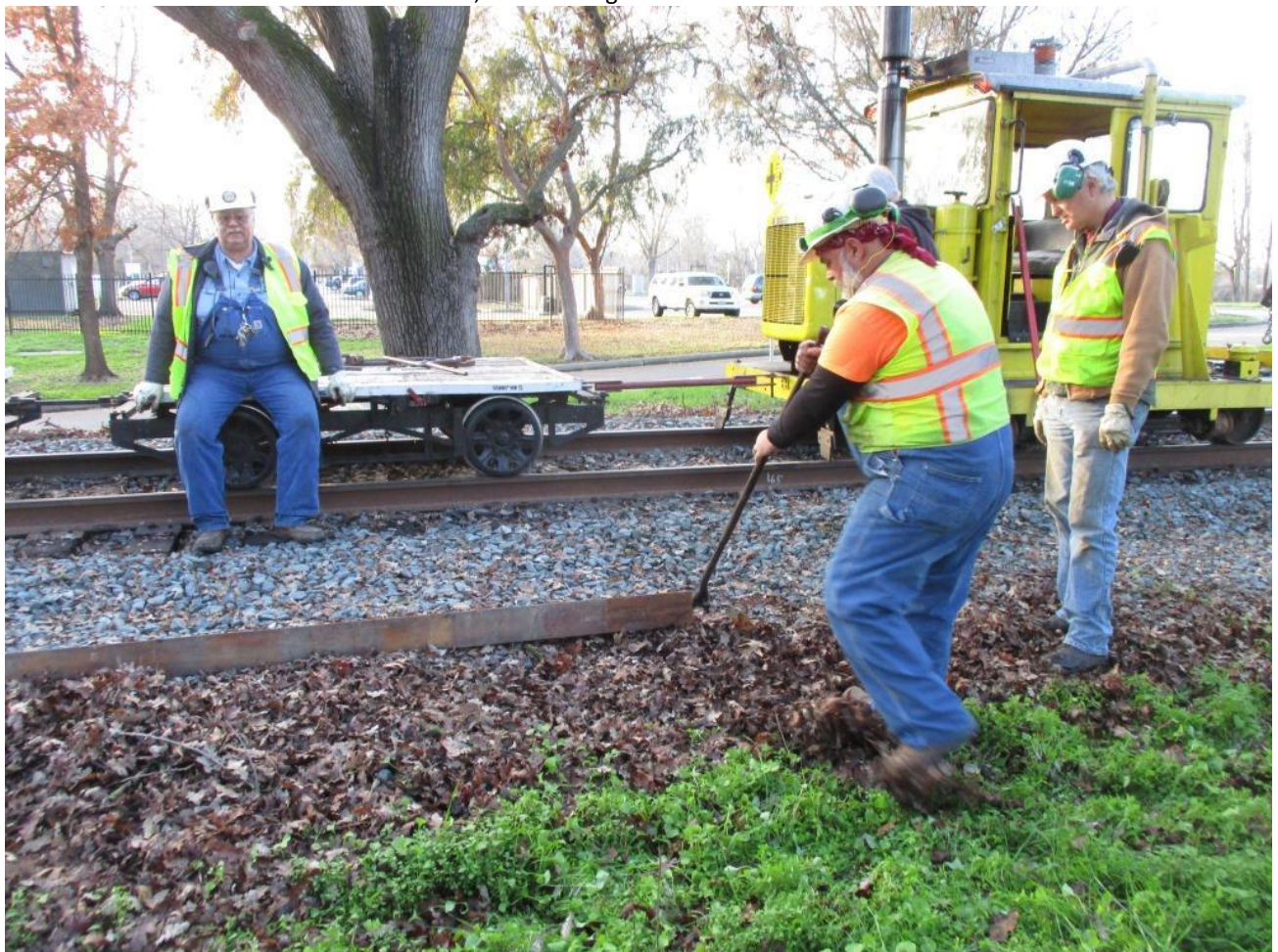
Mike F. uses a rail-fork to roll the rail over to the pile
