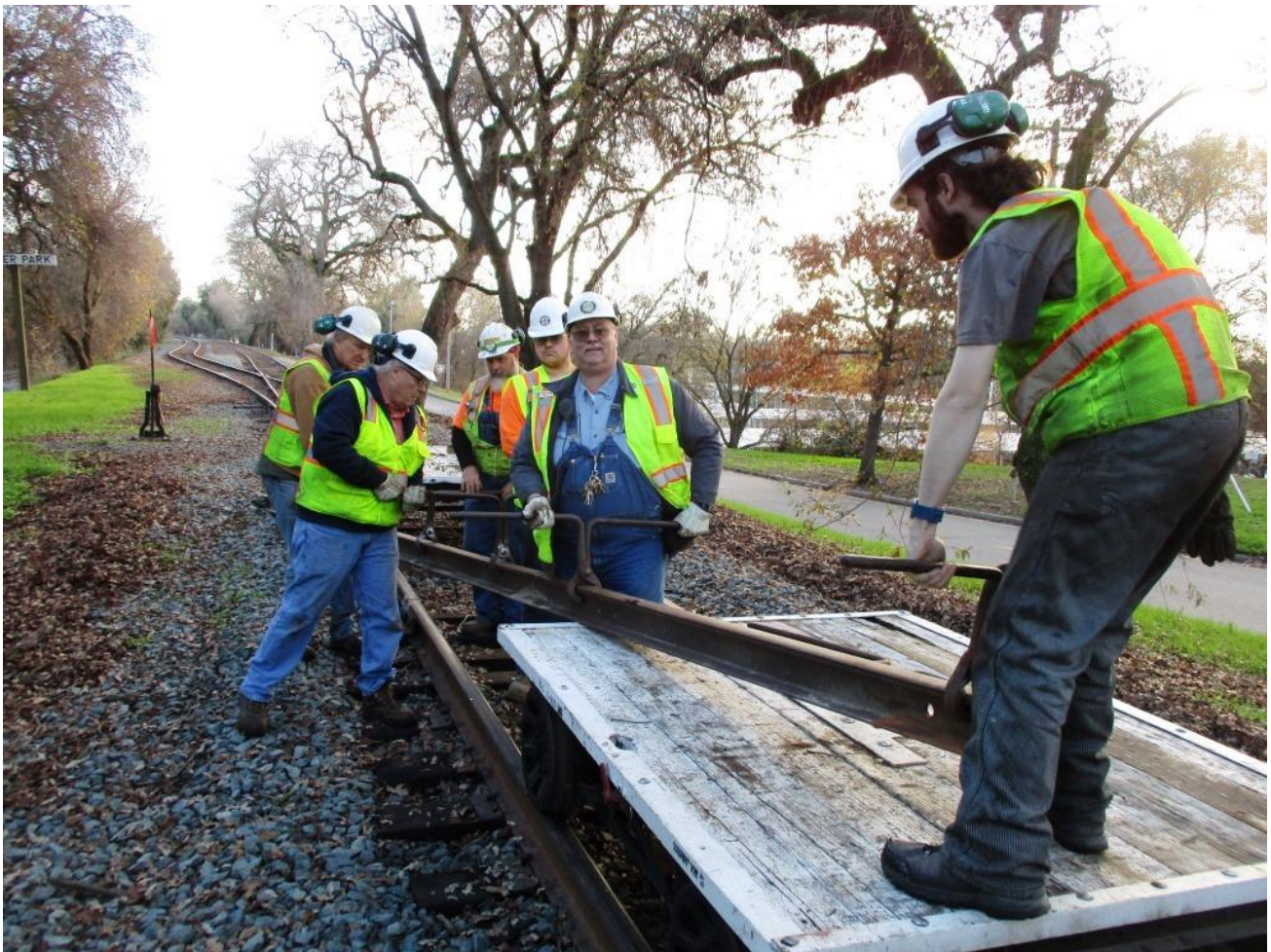
At Front Street, the Team again lifts the rail from the flatcars
