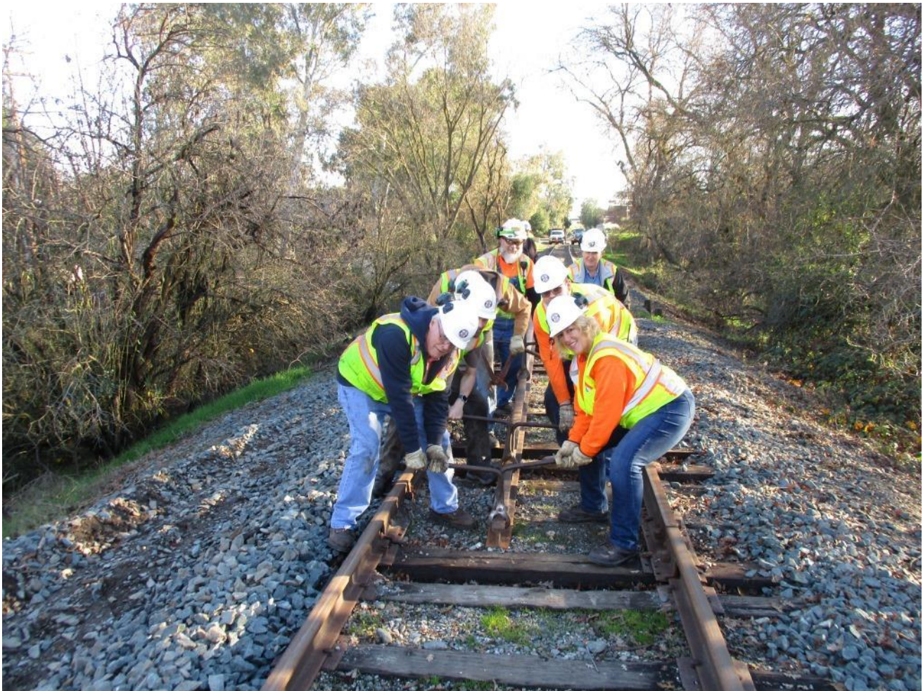
Using two-handed rail-tongs, the Team combines efforts to lift the busted rail onto flatcars
