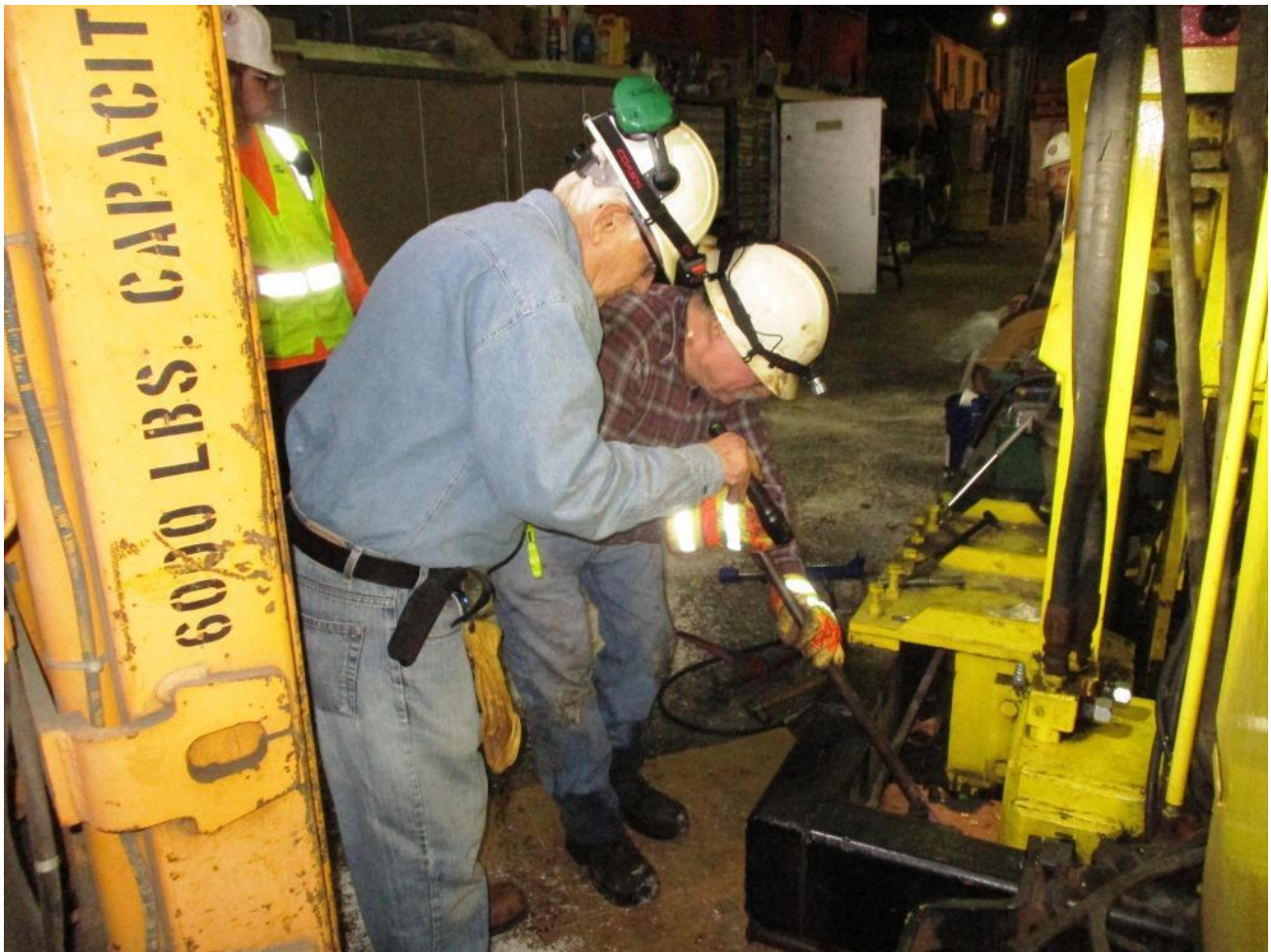
Mike W. and Mike H. pry-out the tie-shear's kicker hydraulic cylinder with a lining bar
